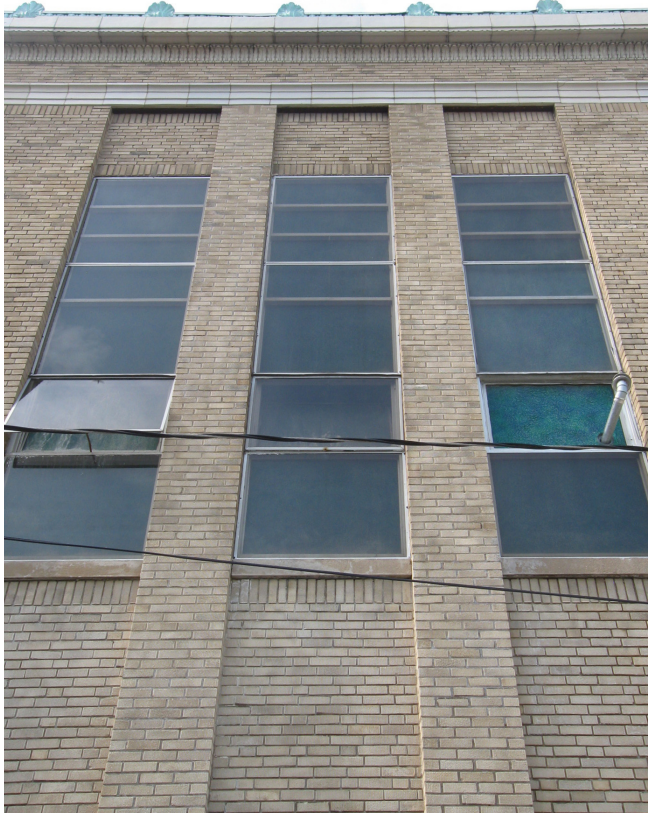
Photo 37. Second floor windows on south facade
