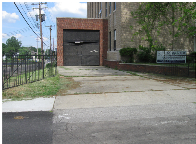
Photo 25. Concrete driveway at north addition
