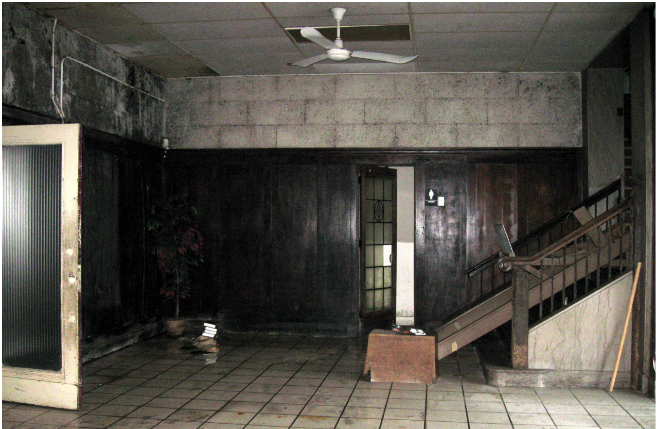
Photo 14. Lobby looking south
