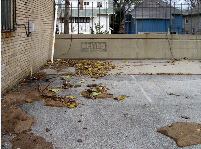
Photo 27. West side of concrete retaining wall
