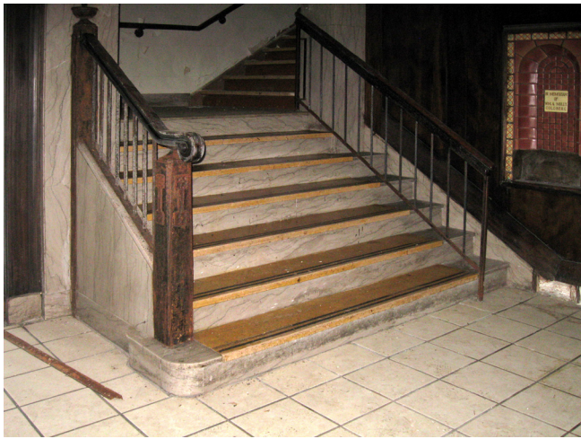
Photo 15. North stairs at lobby
