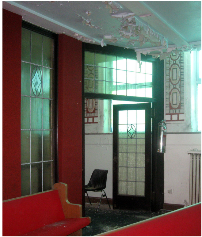
Photo 18. North vestibule doors
