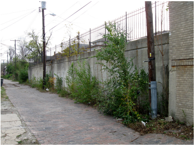
Photo 26. Concrete retaining wall at south parcel
