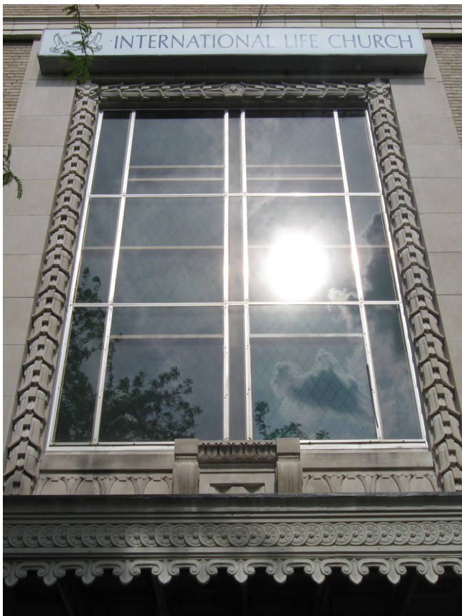
Photo 38. Second floor windows on west facade
