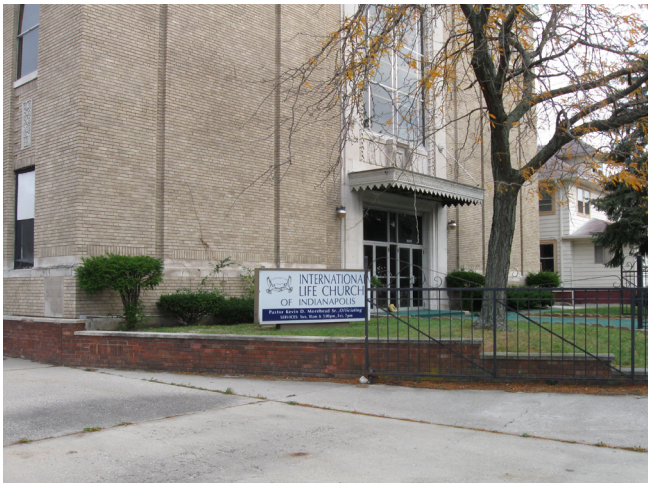
Photo 07. Retaining wall at northern extent
