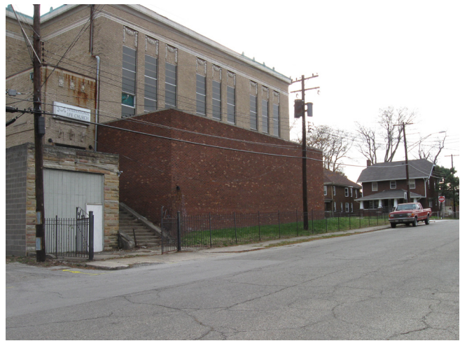
Photo 23. Site at northern extent
