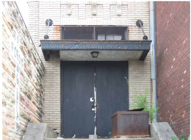
Photo 40. North entry doors and canopy
