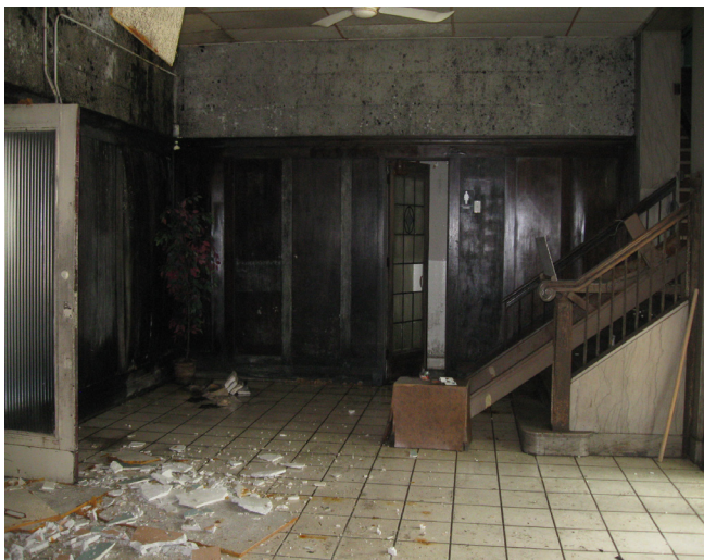
Photo 44. Looking south in lobby
