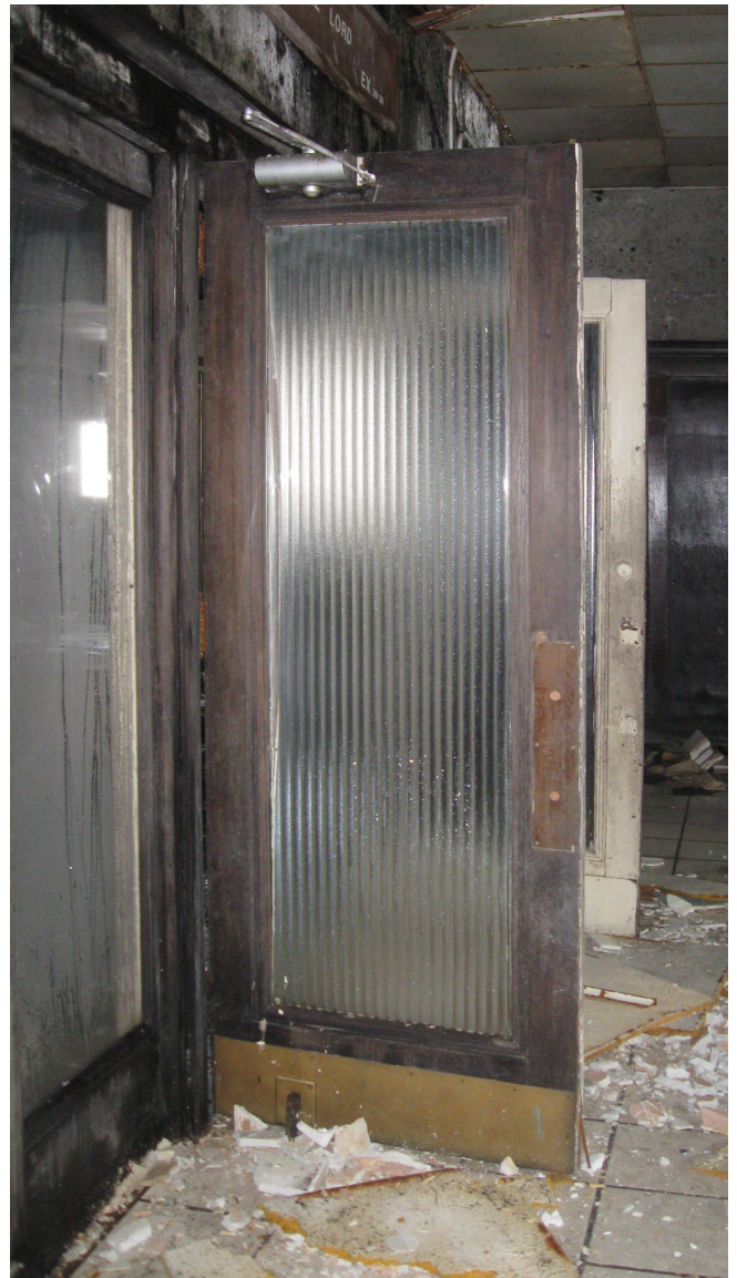
Photo 45. Historic doors in lobby
