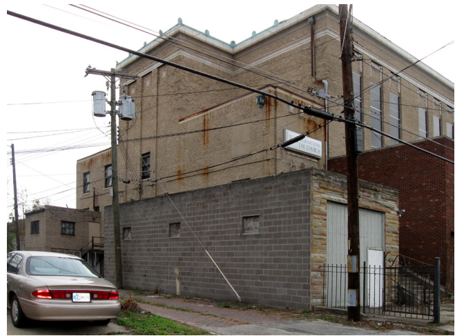
Photo 09. Northeast addition and east facade
