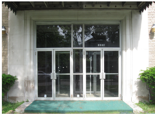
Photo 39. West entry doors
