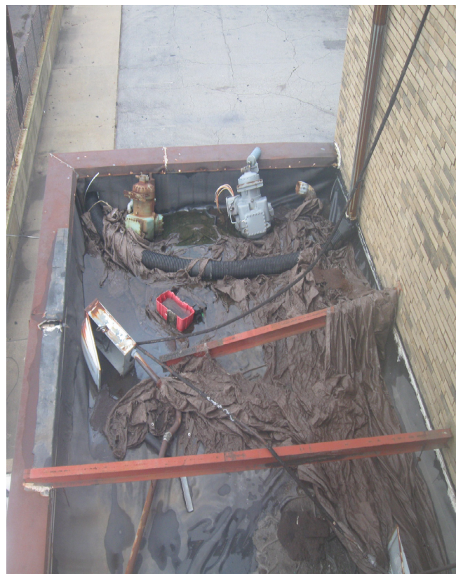
Photo 30. Looking down on Area #3
