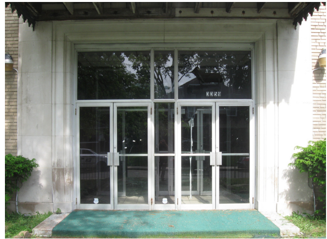
Photo 39. West entry doors
