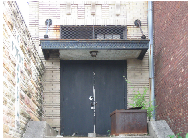
Photo 40. North entry doors and canopy
