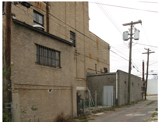
Photo 10. East facade looking north
