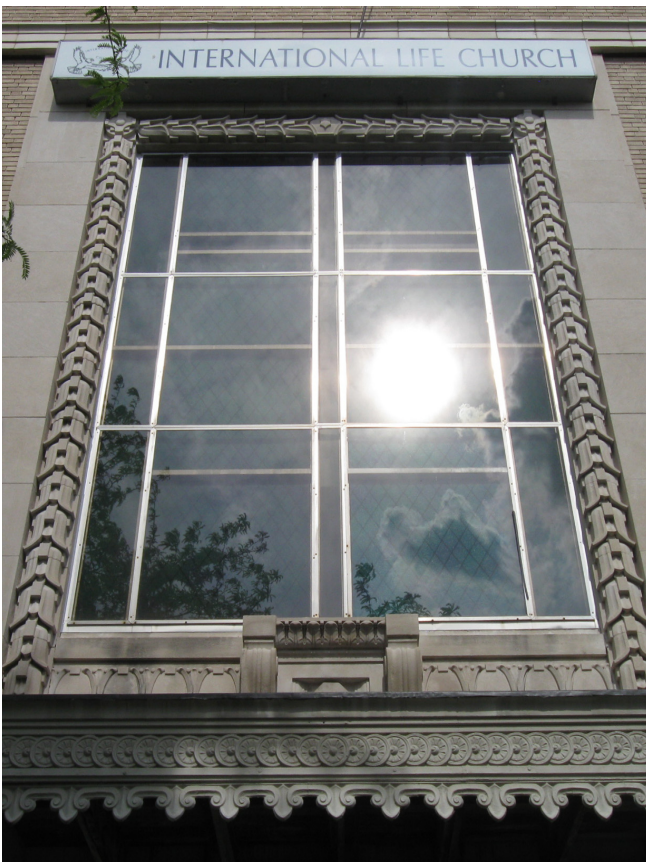
Photo 38. Second floor windows on west facade
