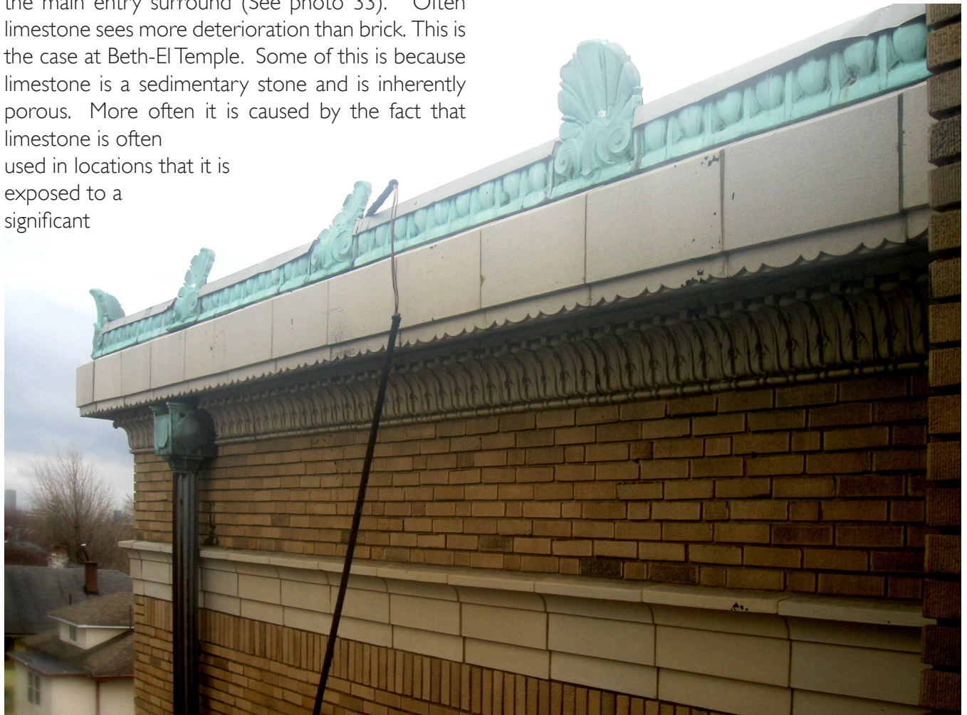
Photo 34. Detail of terra cotta showing out of plane details
