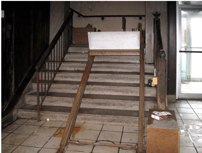
Photo 16. South stairs at lobby
