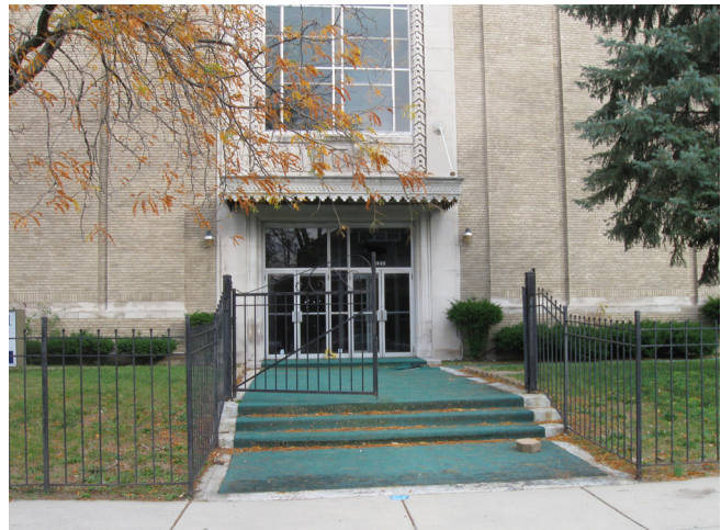
Photo 24. Main entry sidewalk
