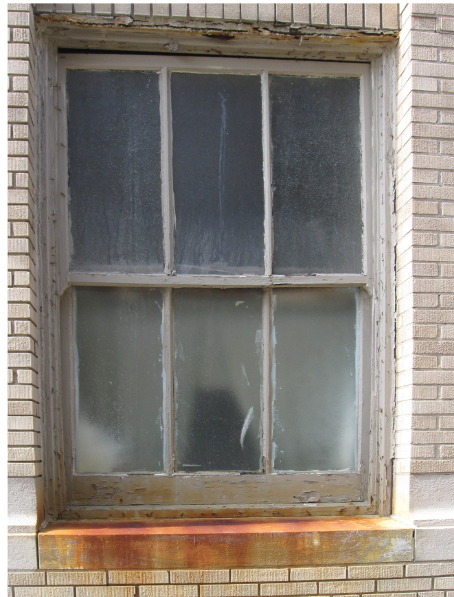
Photo 36. Typical first floor window
