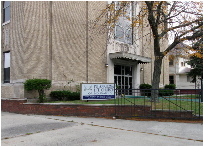
Photo 07. Retaining wall at northern extent
