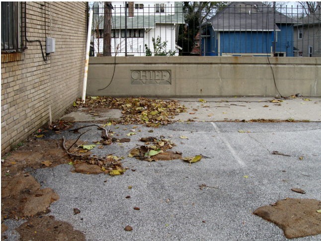
Photo 27. West side of concrete retaining wall
