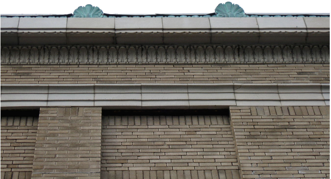
Photo 04. Looking up at terra cotta cornice
