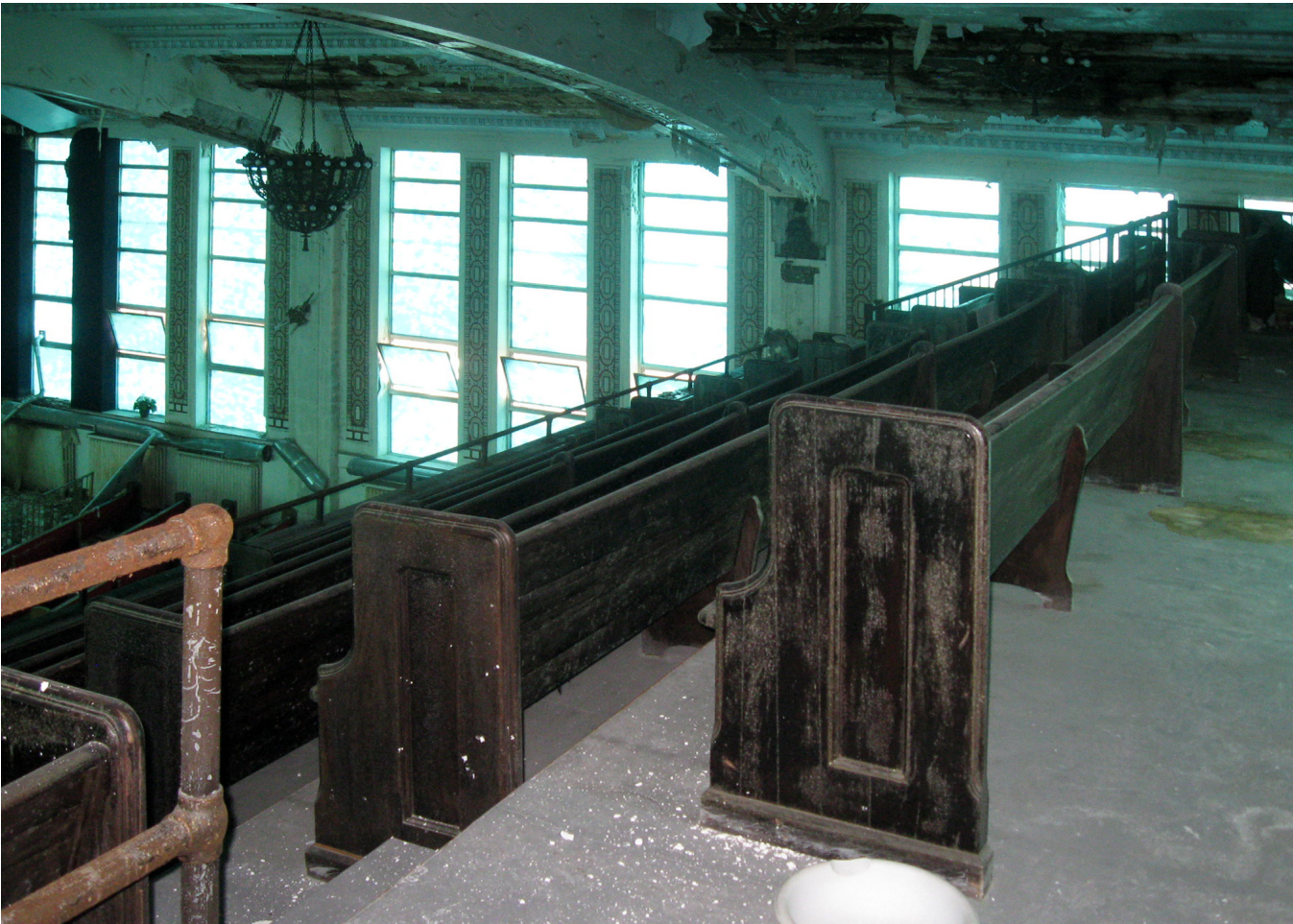
Photo 22. Balcony looking southeast
