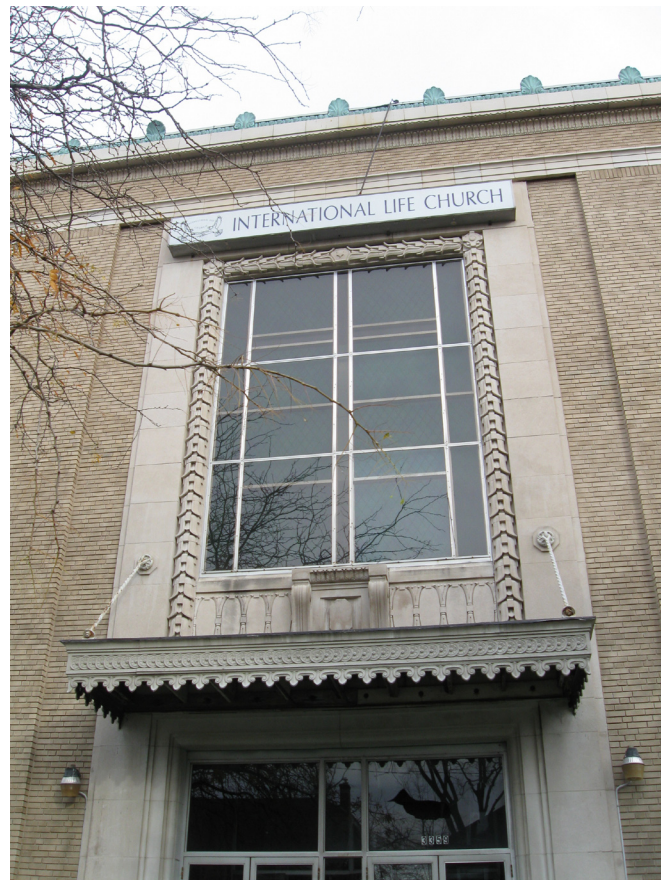
Photo 05. Limestone entry bay with canopy
