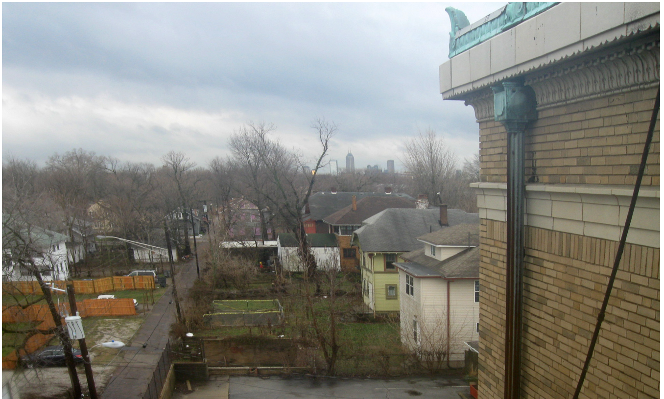
Photo 31. Detail of parapet, conductor head, and downspout
