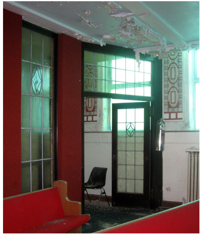
Photo 18. North Vestibule doors
