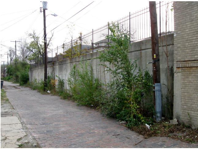
Photo 26. Concrete retaining wall at south parcel
