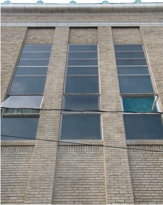
Photo 37. Second floor windows on south facade
