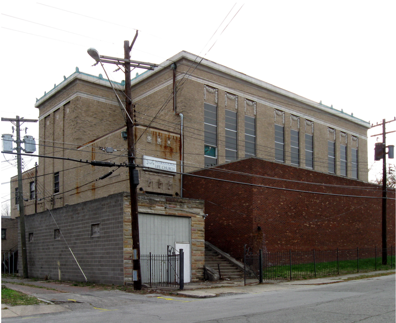
Photo 02. Looking southwest at north facade
