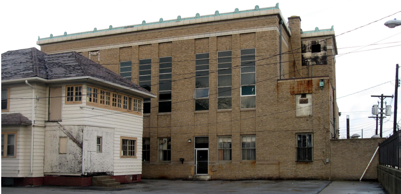
Photo 11. Looking north at eastern extent of south facade
