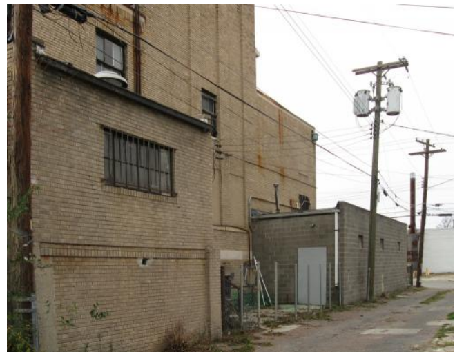
Photo 10. East facade looking north
