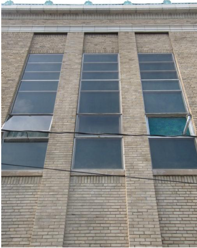
Photo 37. Second floor windows on south facade
