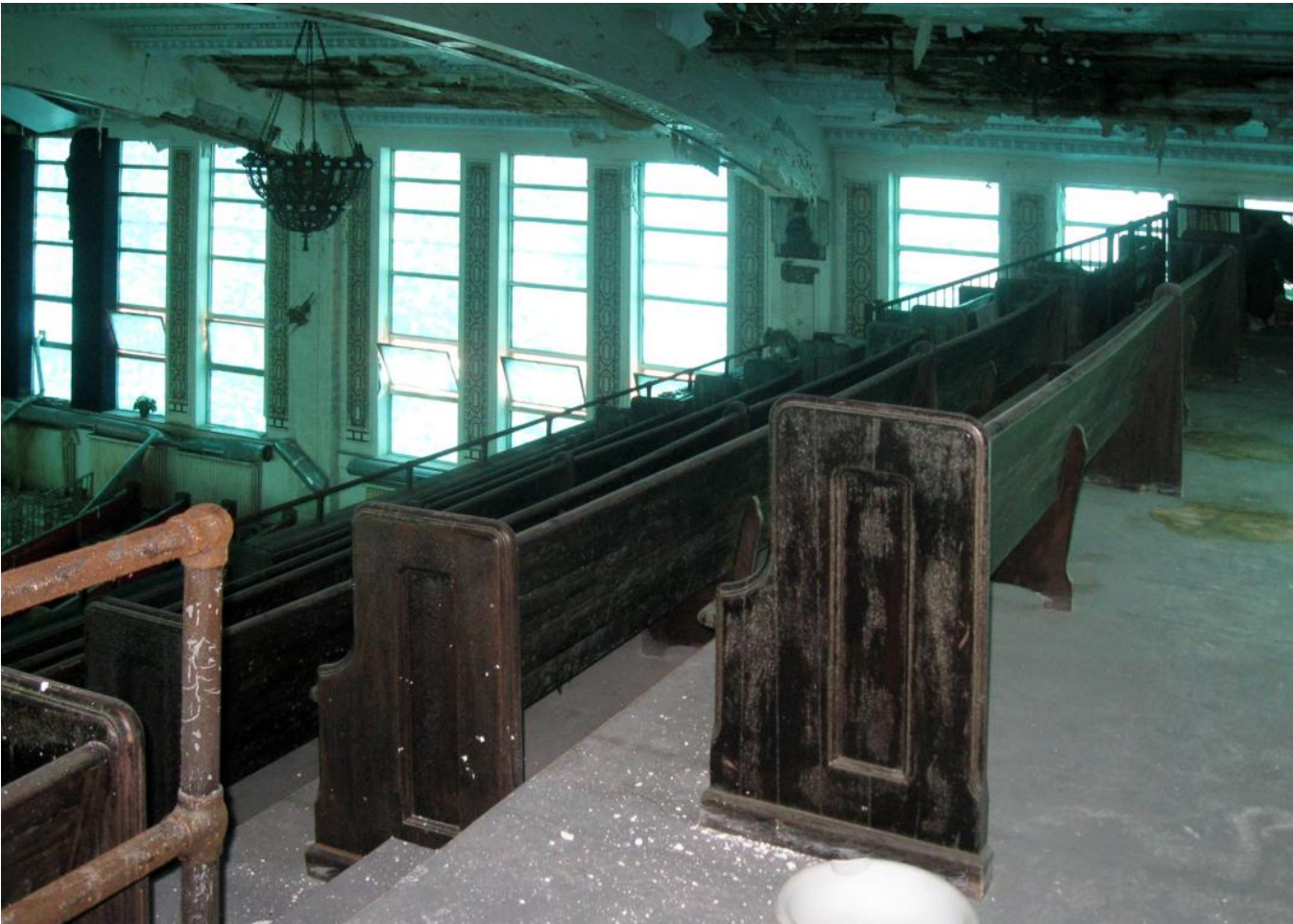
Photo 22. Balcony looking southeast
