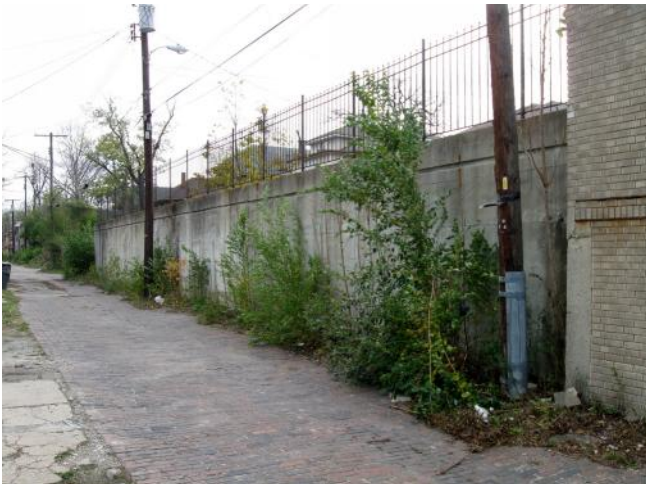
Photo 26. Concrete retaining wall at south parcel
