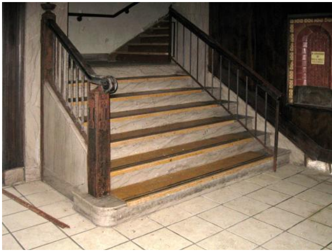
Photo 15. North stairs at lobby
