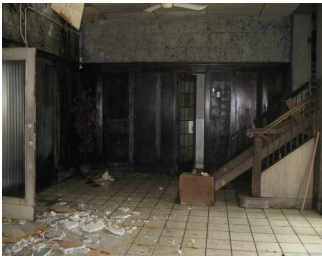
Photo 44. Looking south in lobby
