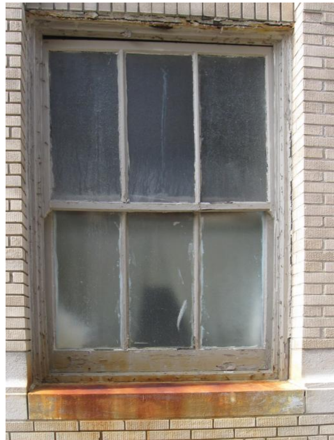
Photo 36. Typical first floor window
