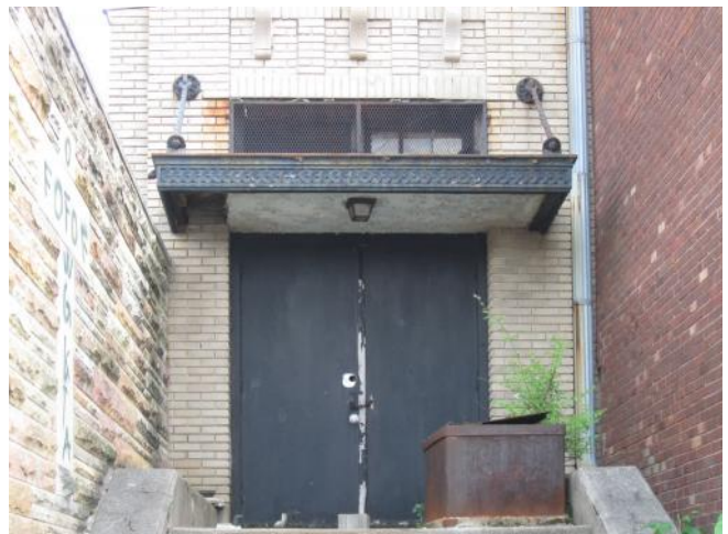
Photo 40. North entry doors and canopy
