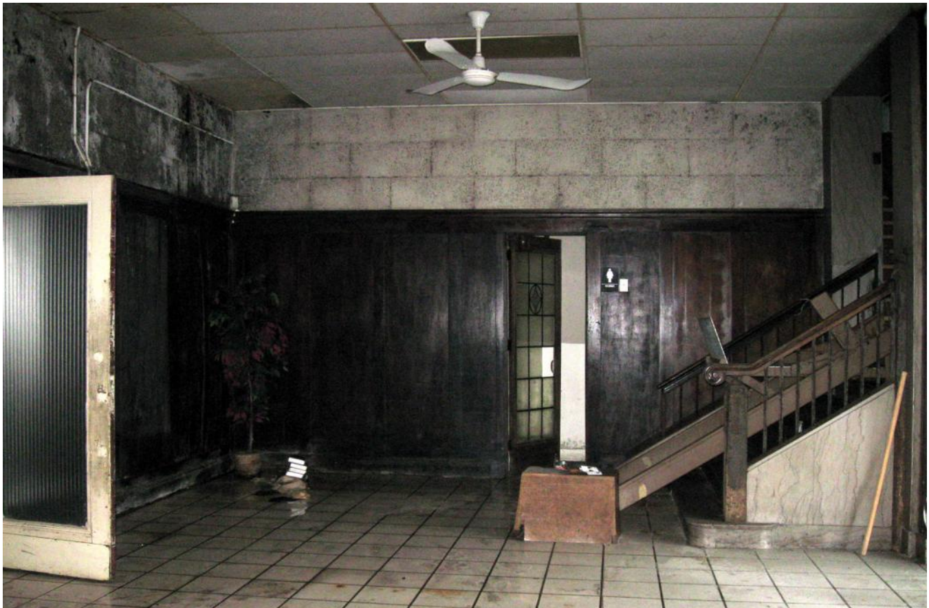
Photo 14. Lobby looking south
