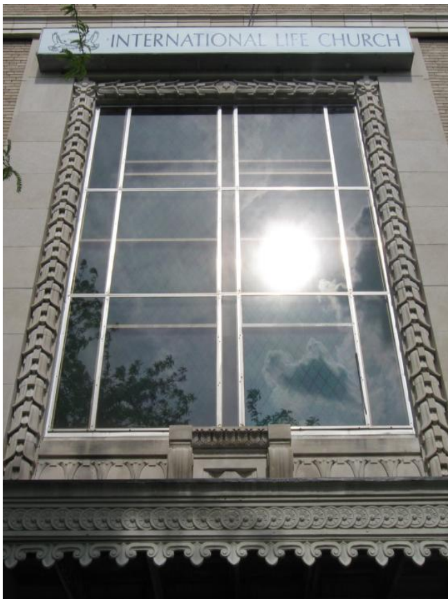
Photo 38. Second floor windows on west facade
