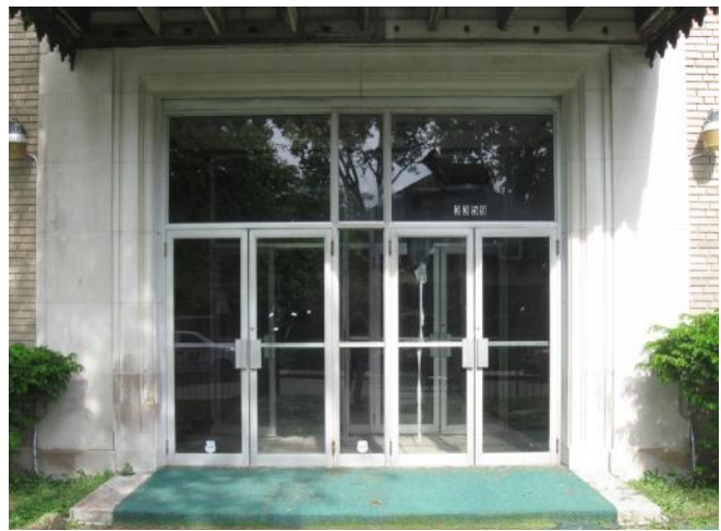
Photo 39. West entry doors
