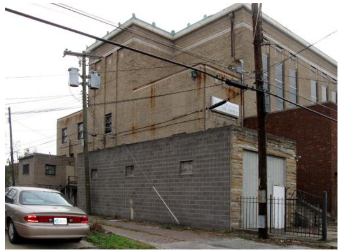
Photo 09. Northeast addition and east facade
