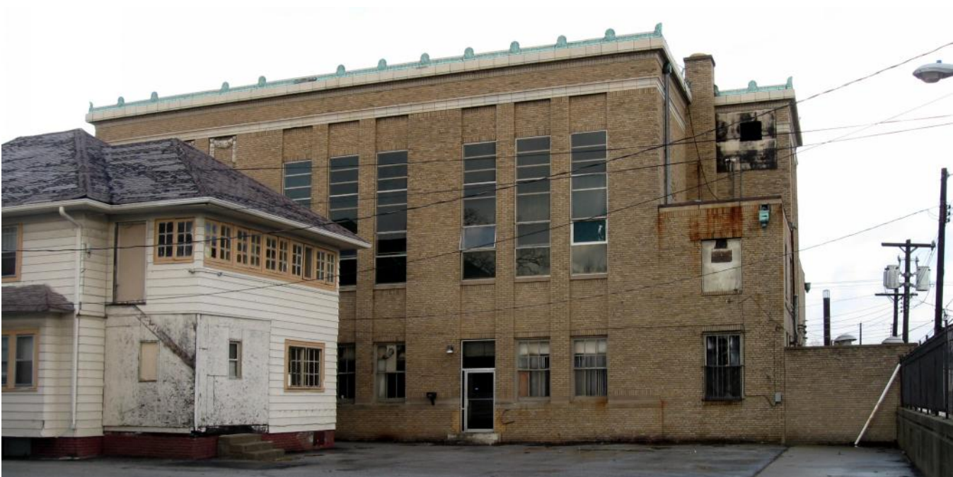
Photo 11. Looking north at eastern extent of south facade
