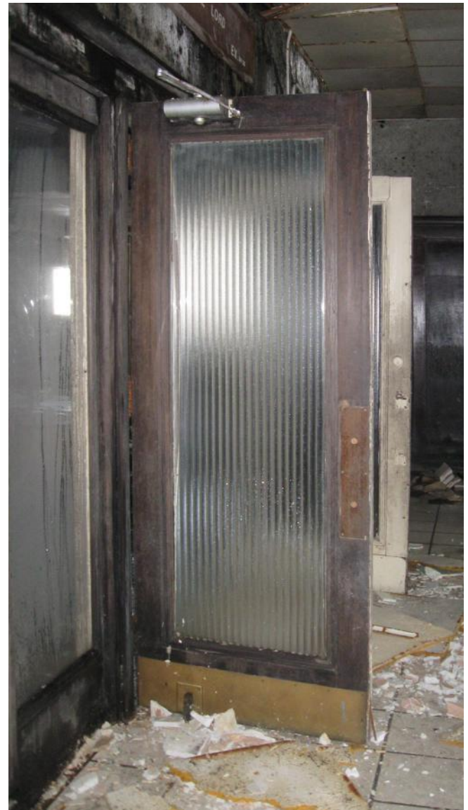
Photo 45. Historic doors in lobby
