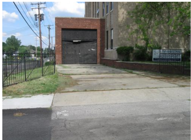
Photo 25. Concrete driveway at north addition
