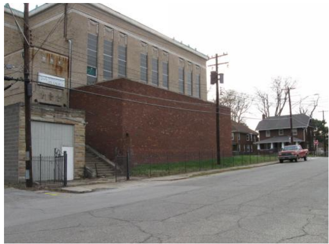
Photo 23. Site at northern extent
