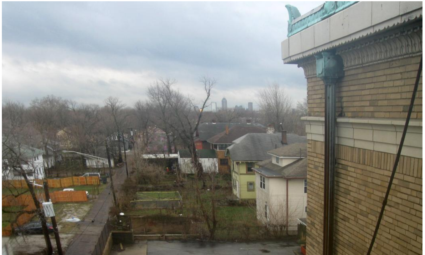
Photo 31. Detail of parapet, conductor head, and downspout
