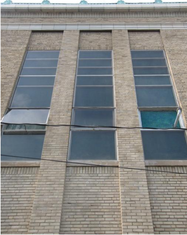
Photo 37. Second floor windows on south facade
