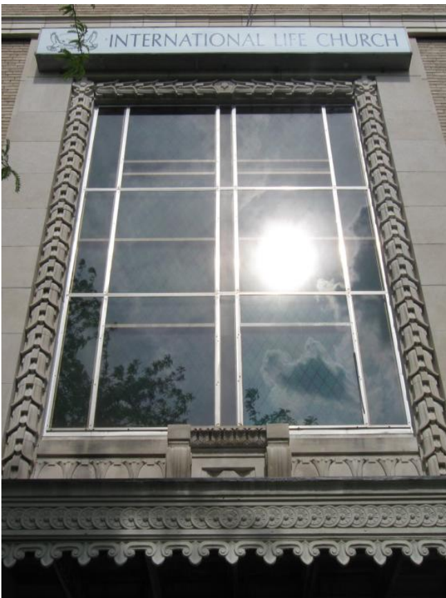
Photo 38. Second floor windows on west facade
