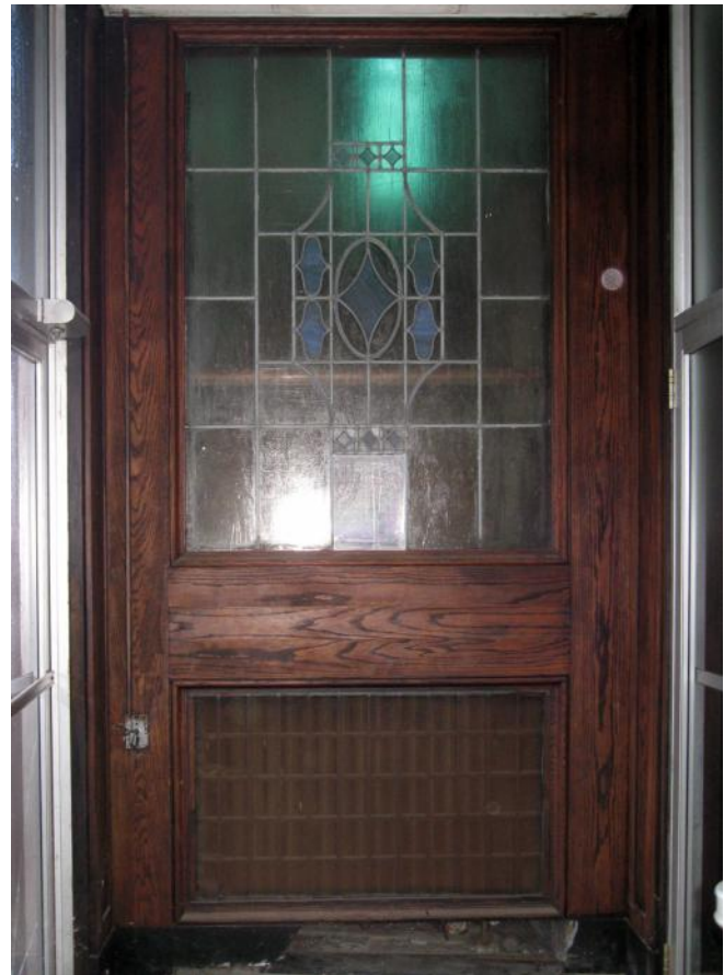
Photo 13. Vestibule wood paneling
