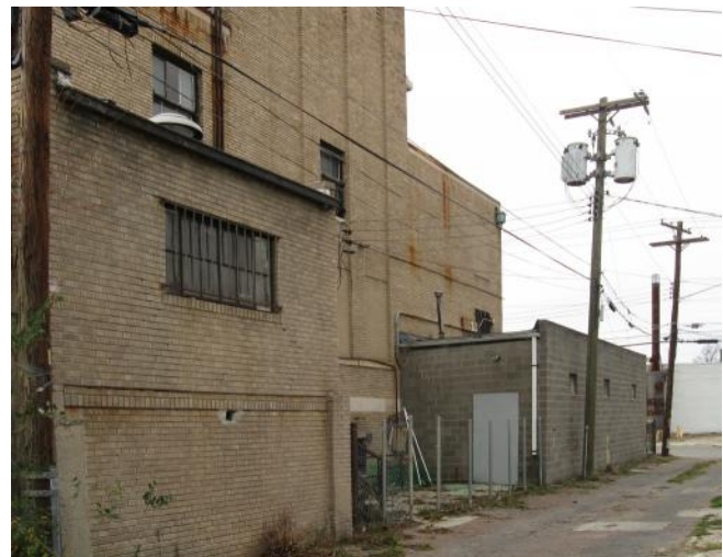
Photo 10. East facade looking north
