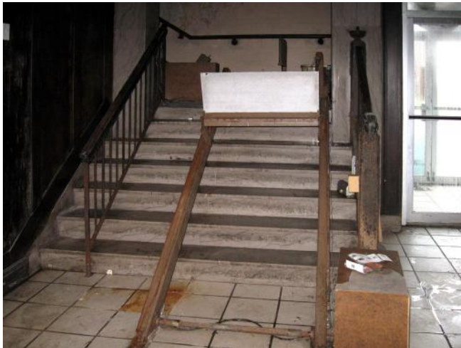
Photo 16. South stairs at lobby
