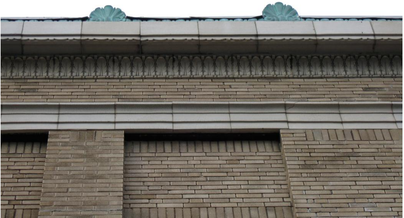
Photo 04. Looking up at terra cotta cornice
