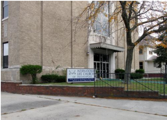
Photo 07. Retaining wall at northern extent
