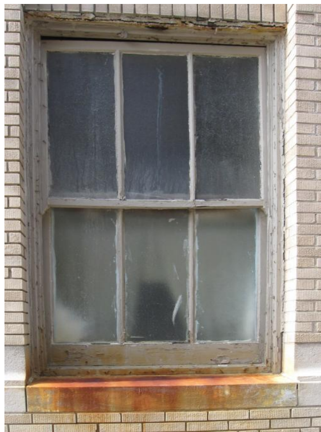
Photo 36. Typical first floor window
