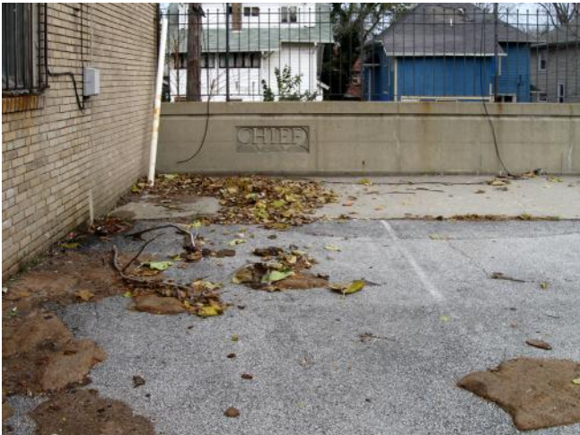
Photo 27. West side of concrete retaining wall
