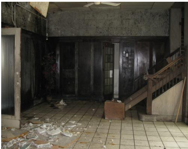
Photo 44. Looking south in lobby
