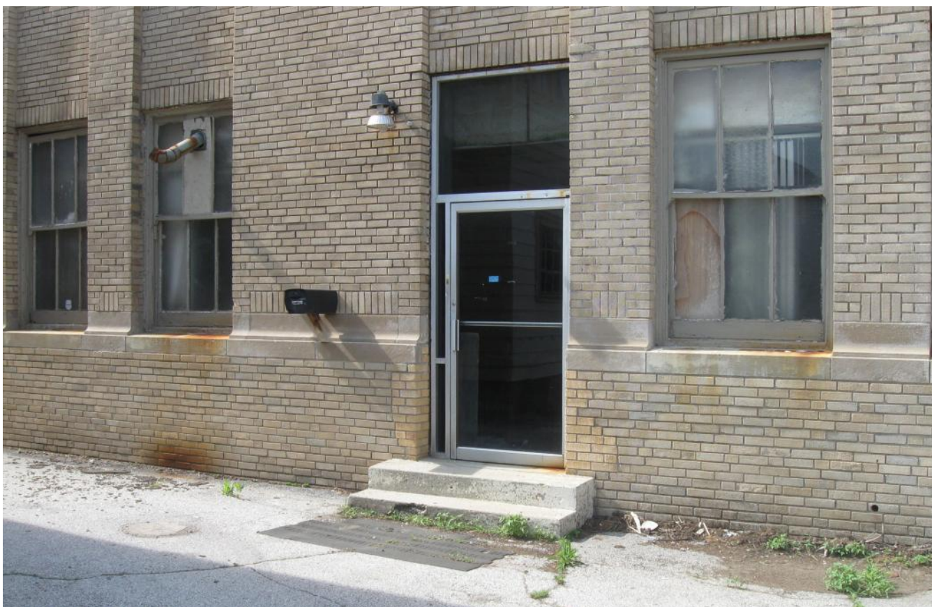
Photo 35. Typical first floor windows and south entrance door
