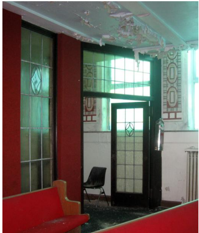
Photo 18. North Vestibule doors
