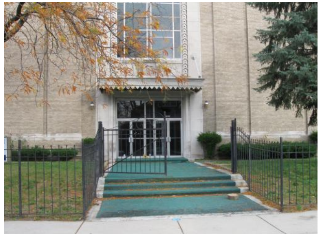
Photo 24. Main entry sidewalk
