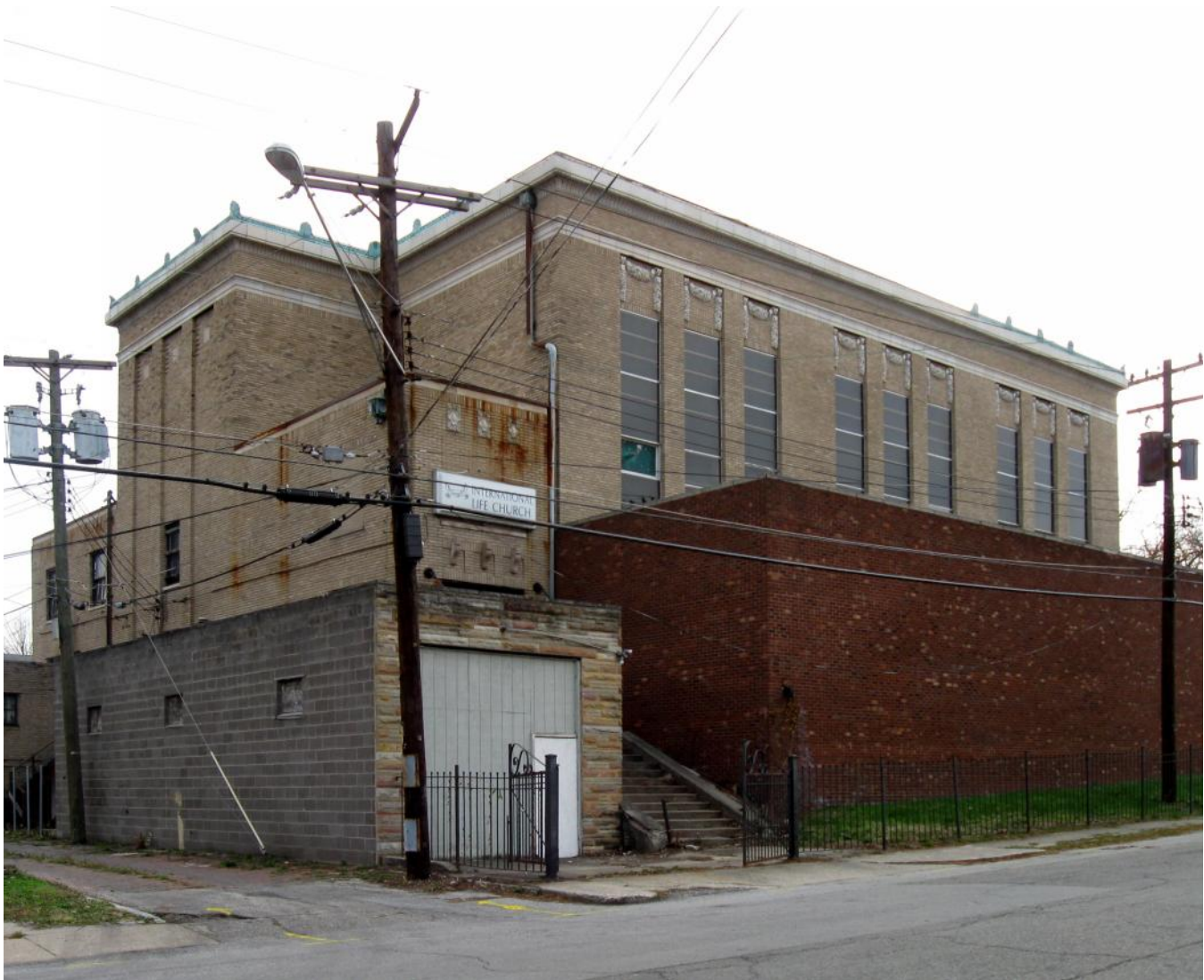
Photo 02. Looking southwest at north facade
